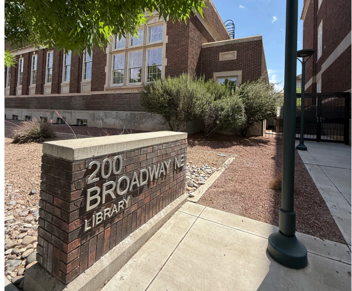
FAT PIPE BUILDING - EXISTING CONDITION
