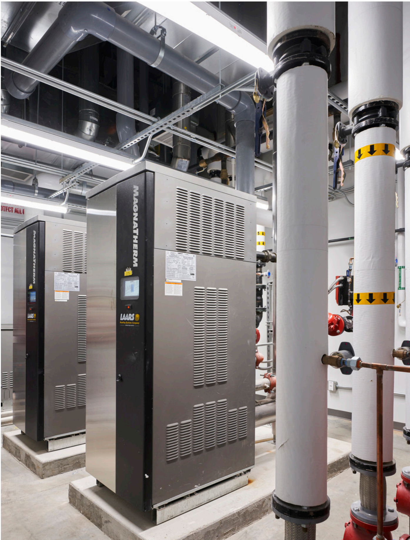
JOHNSON COUNTY MEDICAL EXAMINER'S FACILITY - OLATHE, KS
