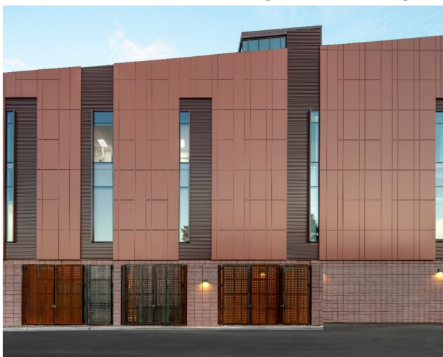
ELECTRICAL YARDS AT THE UNIVERSITY OF ARIZONA APPLIED RESEARCH BUILDING - TUSCON, AZ
